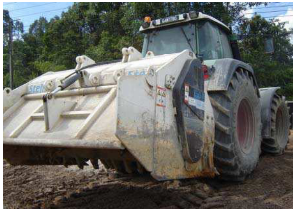
Figure 4 : Sterhr, one of the machinery used in road construction work
