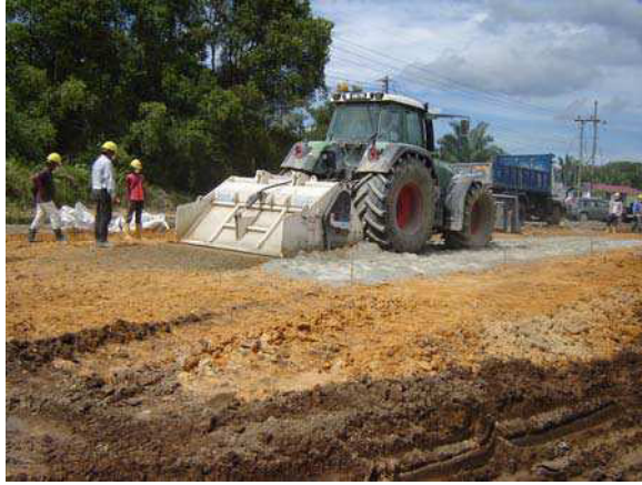
Figure 6 : Mixing process using soil stabiliser machine
