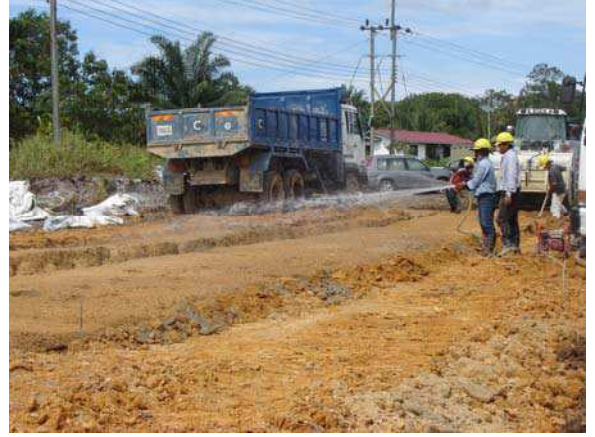
Figure 7 : Spreading water over the road surface.
