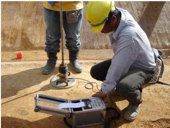
Figure 10 : Falling Weight Deflection Test (FWD) is done in order to determine the quality of product.
