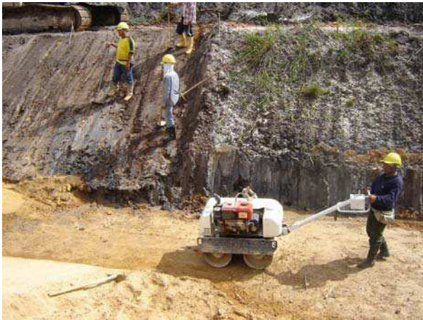
Figure 8 : Manual compaction at site.
