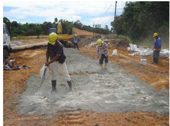
Figure 5 : Spreading cement and GeoCrete mixture along the road to be constructed (manual spreading)
