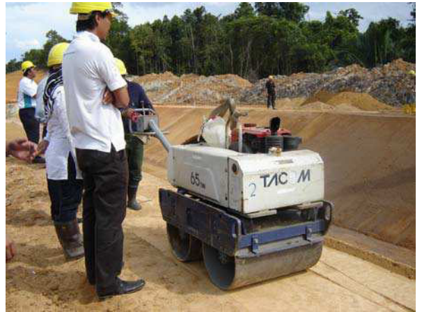
Figure 9 : Vibratory roller for compaction
